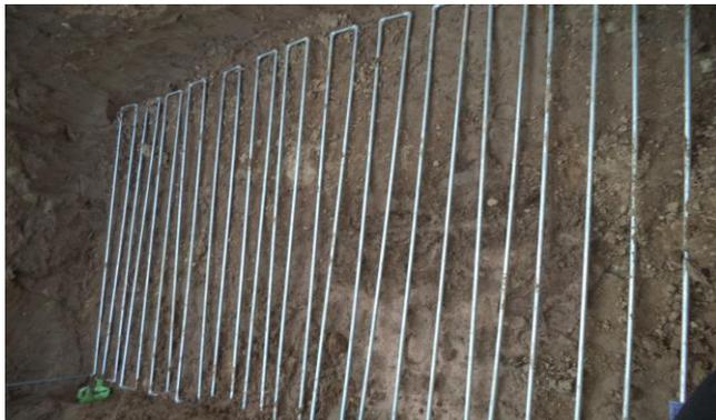
Figure 1: Heat Exchanger (12x14 ft) of Galvanized Iron
